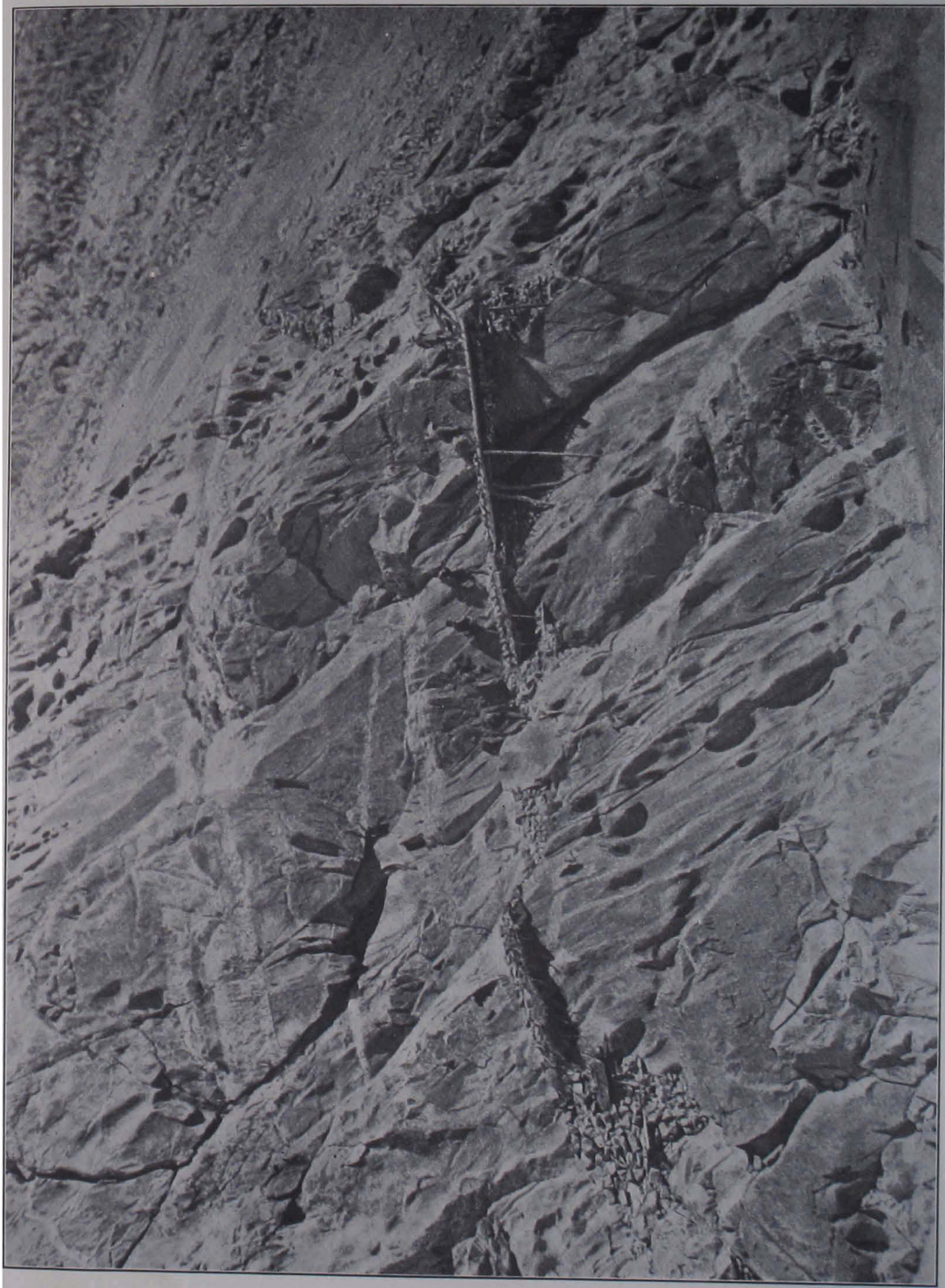
Plate 6. The 'road' on pegs and props north of Hunza.
